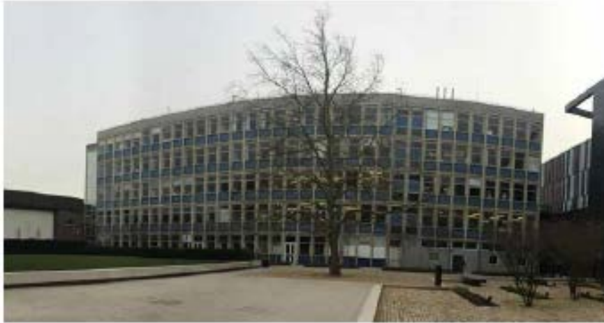
Sinclair Building façade existing
